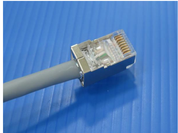
10. Cut the rest tin foil and drain wire.
