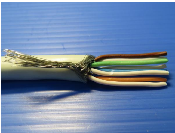
5. Twist the drain wire for welding.
